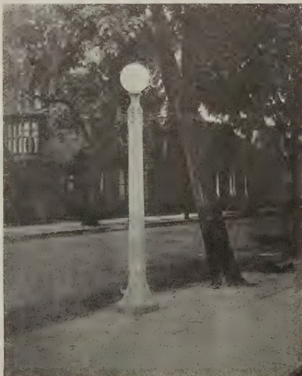
CONCRETE USED TO ADVANTAGE FOR STREET LIGHTING STANDARD
